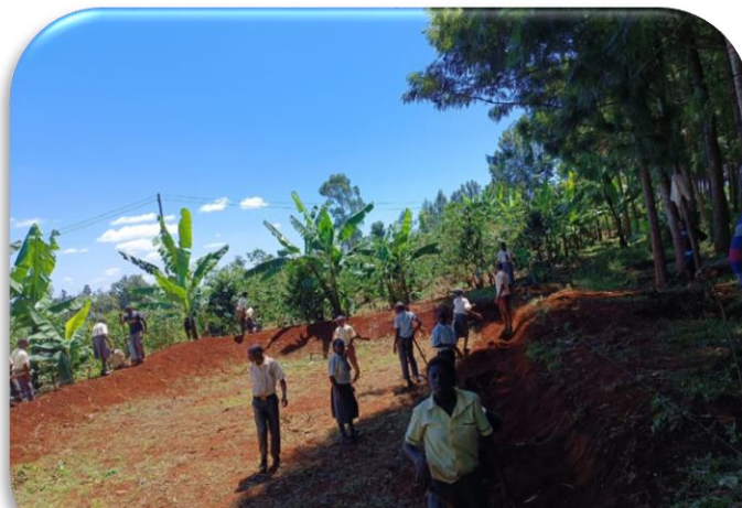
kariru primary pupils participating during pond renovation for pond liner installation.
